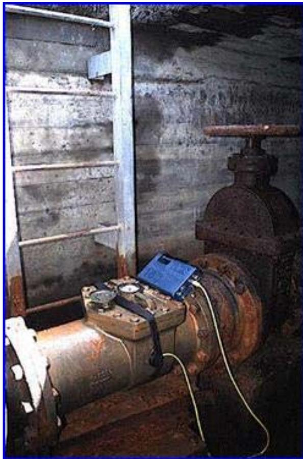
*Figure 2. Data recorder installed on a meter.*
