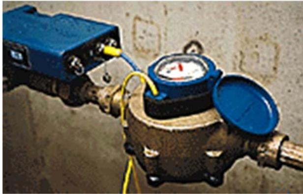
*Figure 1. Data recorder installed on a meter.*
